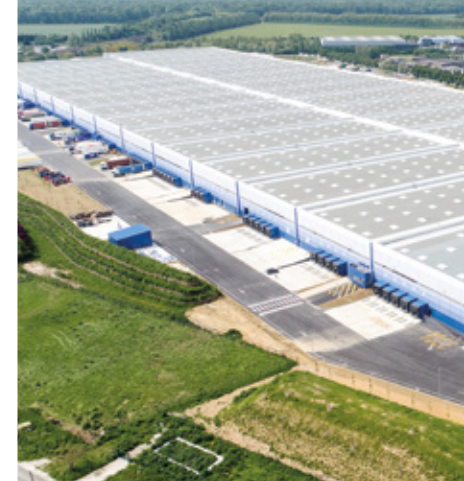
ARGAN / GAZELEY | ALMACÉN SECO | 200 000 M 2 | TOUR
